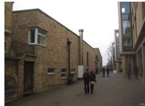
Existing Library facade to Christ's Lane
