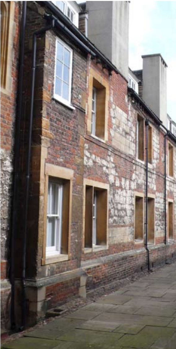
Potential to incorporate historic wall of First Court range
