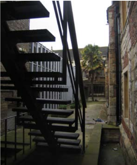
Existing view showing external staircase and many level changes.
