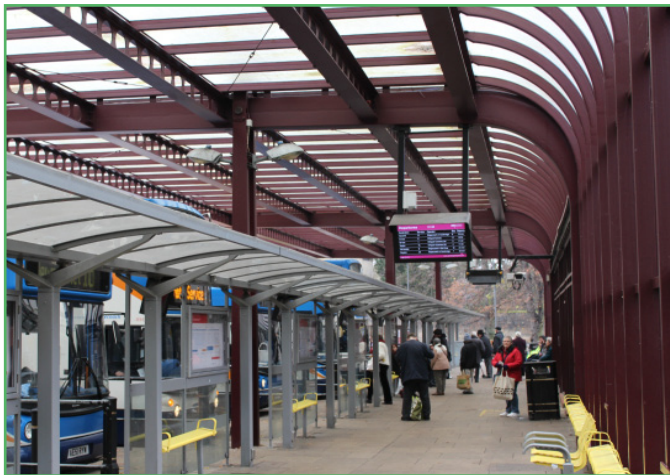
Canopy detail to Cambridge Bus Station
