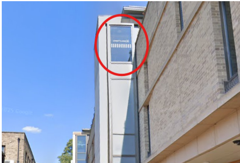
Figure 3: Photo illustrating window 39 extending to upper floor level
