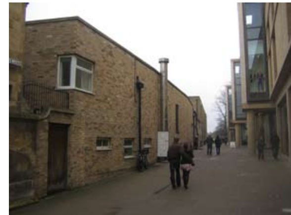
Existing Library facade to Christ's Lane
