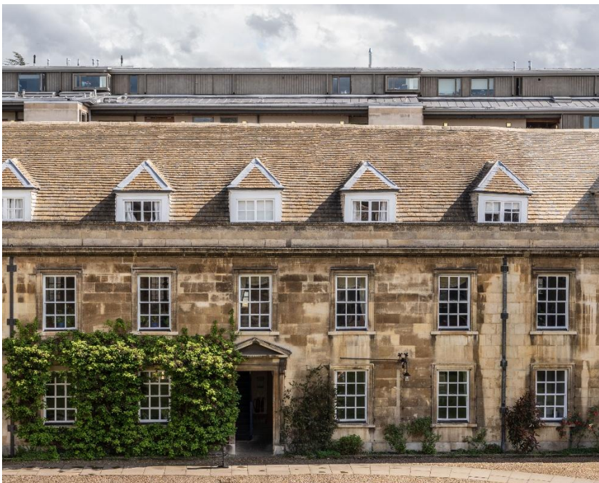
Looking south from first floor rooms in Entrance Court – the College's Grade I Listed Buildings with the apartments in the development on the south side of Christ's Lane seen behind.
