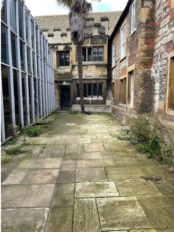
From left to right, the present library, the Bodley Library and First Court (south elevation) showing the proximities and poor quality of space.
